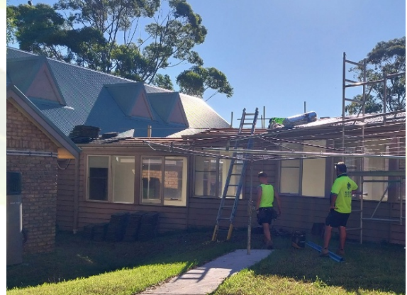
The latest section of new roofing taking shape.
